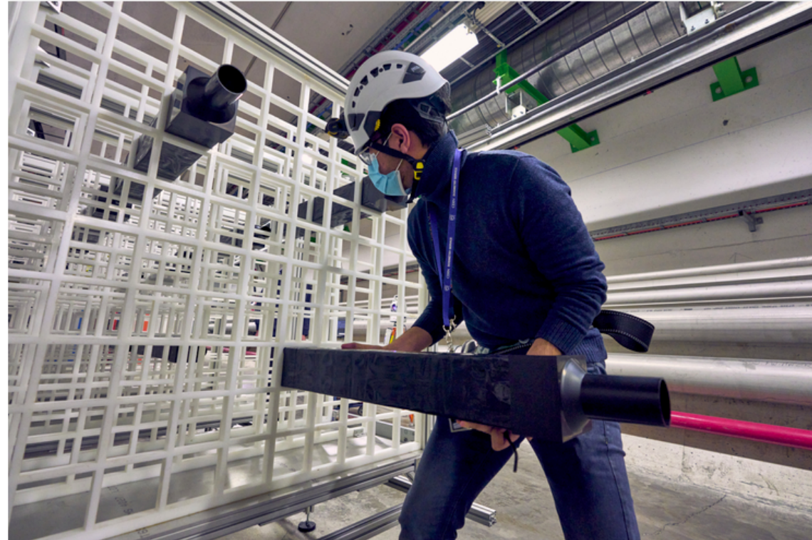
Installation of the support structure for the MAPP detector components. (Image: CERN)
